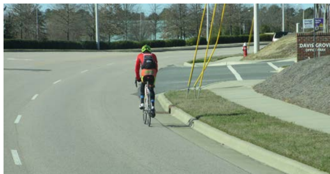
Wide outside lanes on Davis Drive
