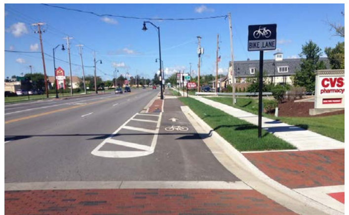
Separated bike lanes with a raised median as vertical separation (Not currently in use in Cary)
